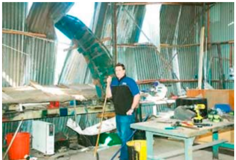
The long strip of container lodged in the wall was thrown several hundred metres and through the wall of the shed.
